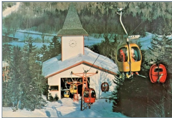
Gondola 2 Base Station;
